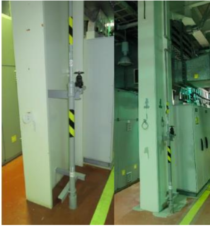
Figure 5. Pillars reinforcement (before and after)
