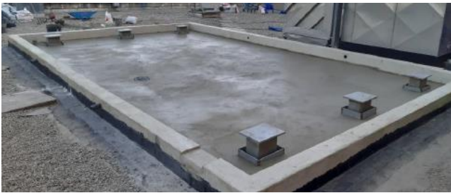
Figure 6. New Unit basement
