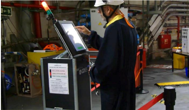
Figure 1. Vigia System at Cofrentes NPP.
