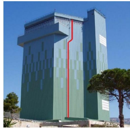
Photography 2. Exterior appearance of the Weather Protection Building
