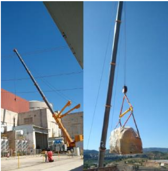
Figure 7. New Unit lifting
