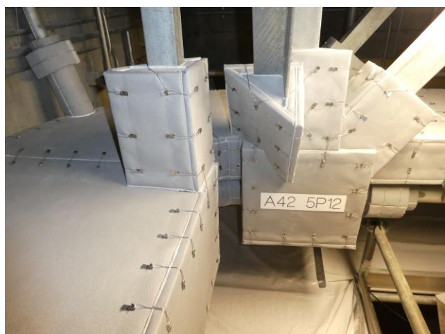
Figure 1. Darmatt KM1 passive protection installed by GDES Auxiliary +108 Vandellós II NNP (Spain)
